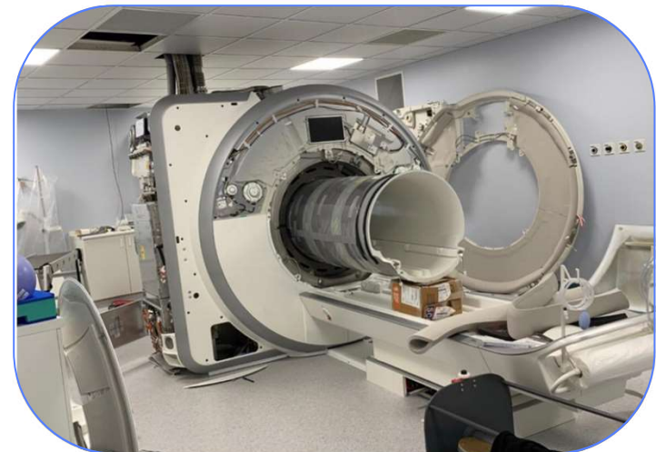
2020 installation of 1.5T scanner in Stracathro
