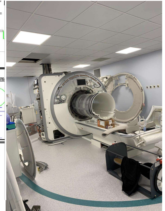
2020 installation of 1.5T scanner in Stracathro
